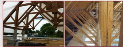
The left image is an example of exposed structure while the right image is an example of unexposed structure in the mezzanine.
